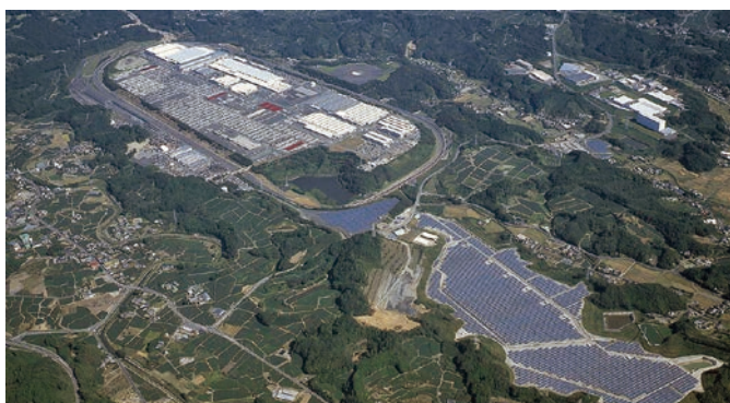
Suzuki Makinohara Solar Power Plant
